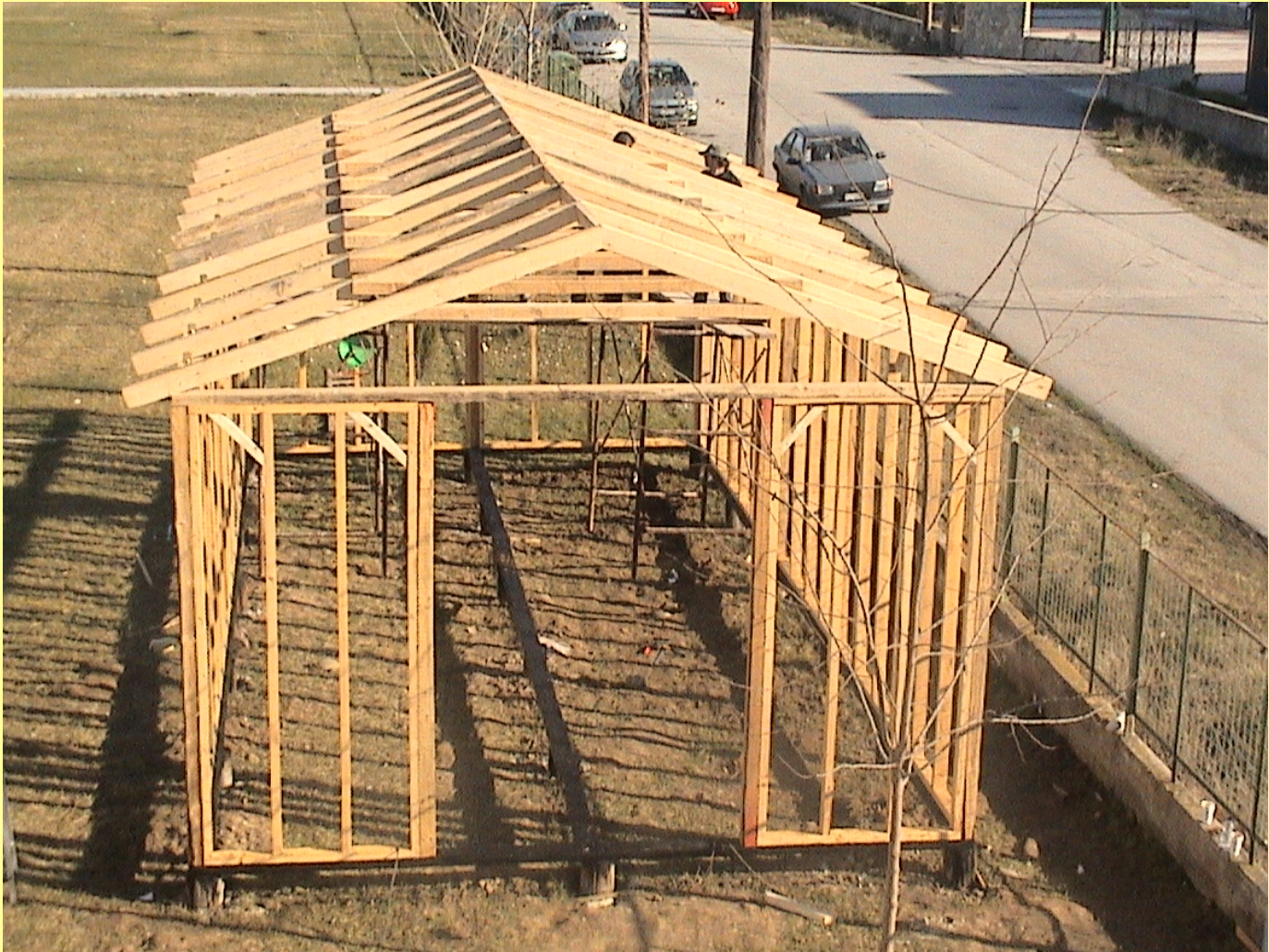
Roof construction from prefabricated elements The complete wall and roof skeleton
